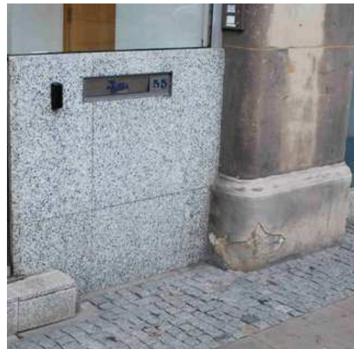
2. Facing stones made of grey granite and sandstone, Halifax Bank, Sheffield. (Photos: Peter Kennett)
